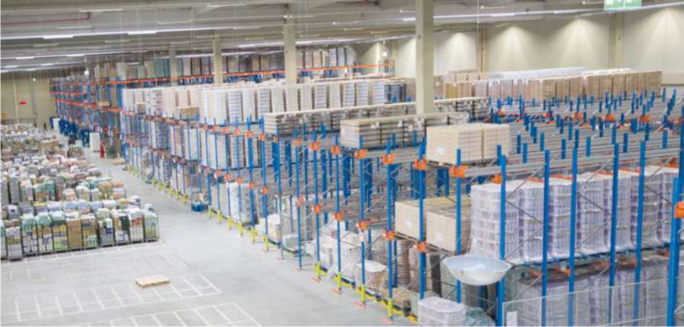
Shuttle warehouse with inclined roller track
