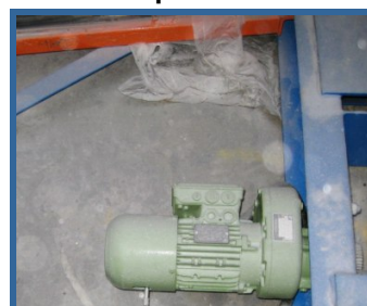
Serious damage can be caused by loose shrink wrap left lying on your coldstore floor.
