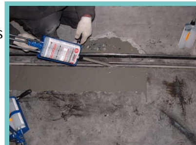
Spalpro being applied to floor
