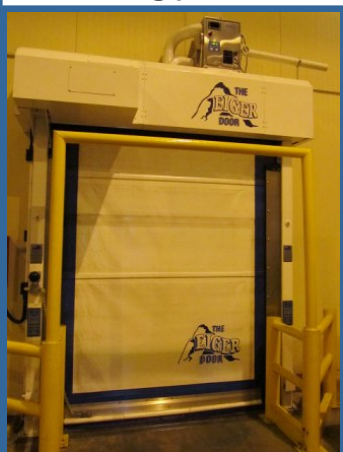
An Eiger door with a dehumidifier above.
