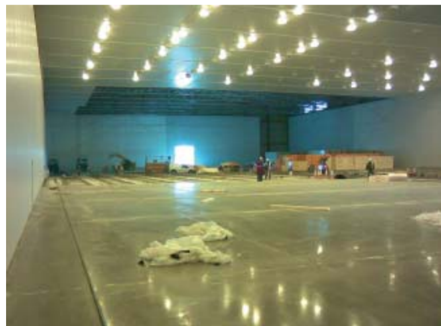
New chamber under construction at Reed Boardall.
