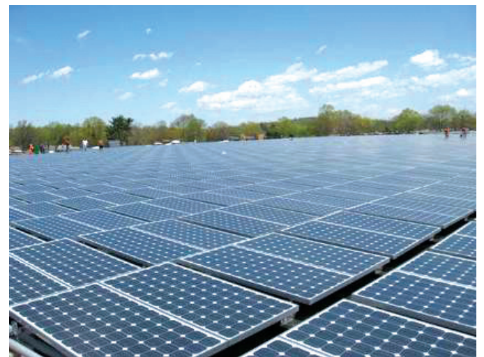
Photovoltaic cells on the roof of Halls Warehousing in the US.
