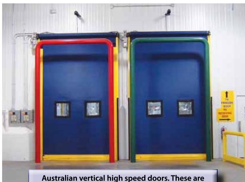
Australian vertical high speed doors. These are now insulated and do not require solid night doors
